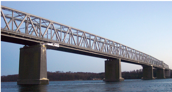
Ponte 'The Little Belt', Dinamarca
